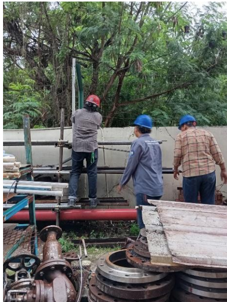
Gambar 3. 3 Install Unit CCTV
