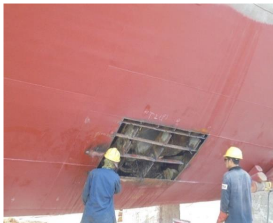
Gambar 2.21 Repleting plate area bottom
