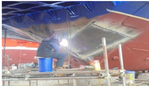
Gambar 2.14 Repleting plate area bottom
