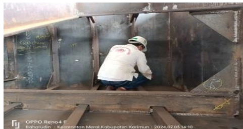
Gambar 2.5 Inspect double bottom
