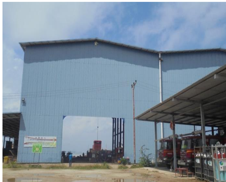
Gambar 1.4 Main wokshop fabrication
