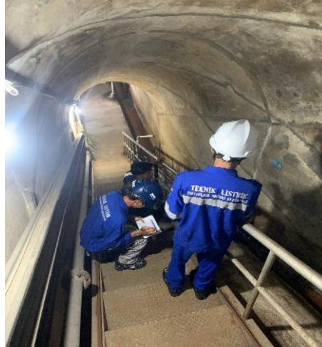
Gambar 3.57 Mengukur nilai di dam galery
