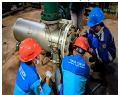
Gambar 3.5 Pembersihan filter stainer
