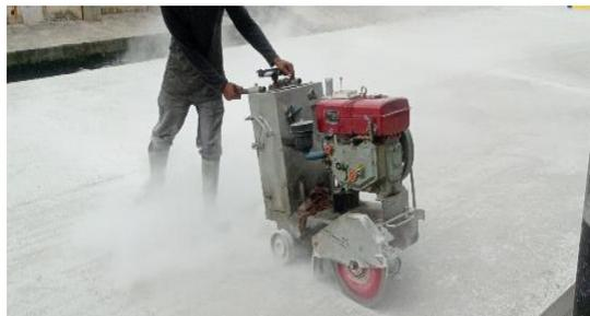
**Gambar 3. 9 Mesin Cutting Rigid**
