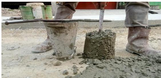
**Gambar 3. 28** Uji Slump
