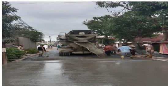
**Gambar 3. 35** Pengecoran Beton
