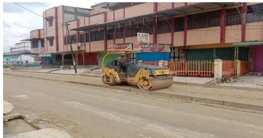
**Gambar 3. 4** *Vibration Roller*
