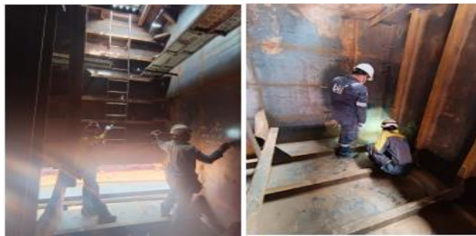
Gambar 3.16 inspection with class Sumber : Penulis
