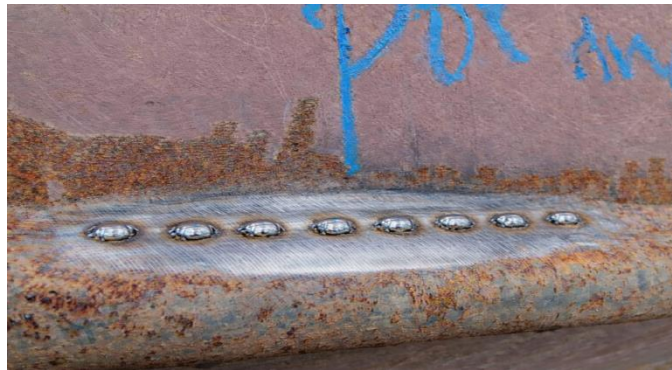
Gambar 4.3 Defect Porosity In Tack Weld
