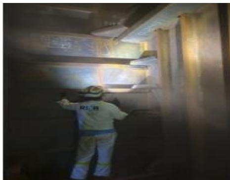
Gambar 3.11 inspection with class Sumber : Penulis
