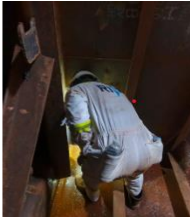
Gambar 3.14 inspection with class Sumber : Penulis
