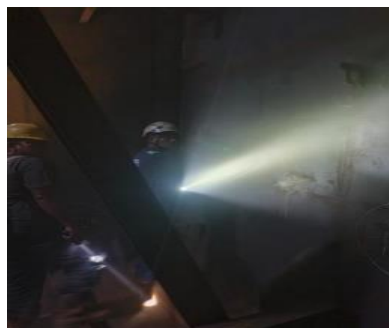
Gambar 3.5 Inspection with class Sumber : Penulis
