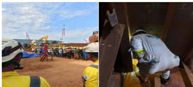
Gambar 3.8 Breefing general & inspection with class Sumber : Penulis
