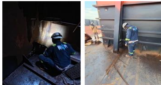
Gambar 3.12 inspection with class Sumber : Penulis
