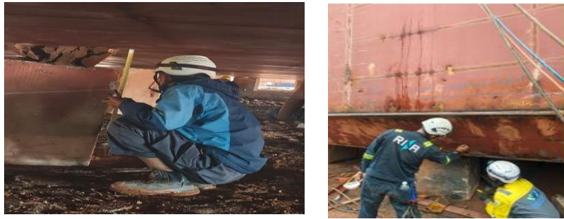
Gambar 3.7 pengambilan keel deflection & inspection with class Sumber : Penulis
