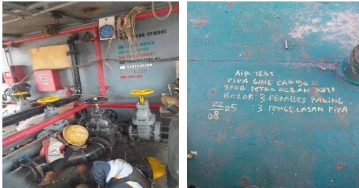
Gambar 3.29 Air test SPOB PETRO OCEAN XVII
