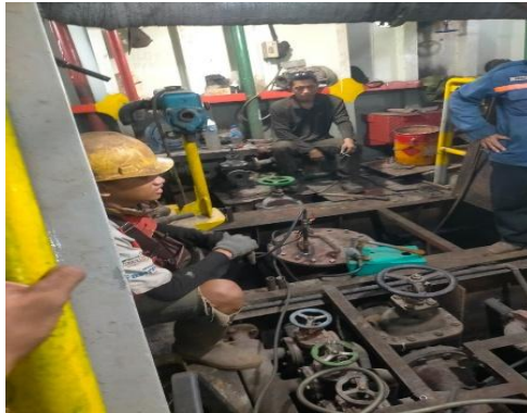
Gambar 3.49 Hydro Test TB TSE 3
