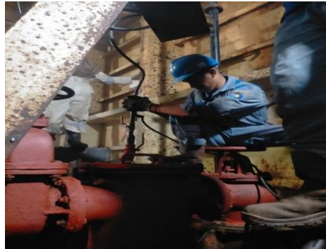
Gambar 3.36 Hydro test valve sea chest
