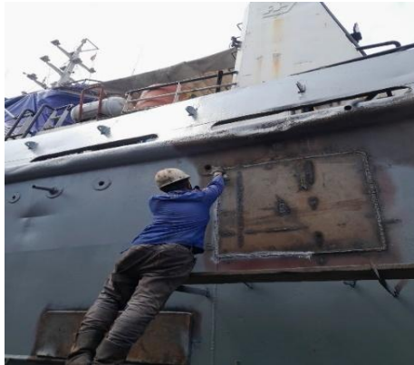
Gambar 3.82 Penetrant test TB.MARINA 22
