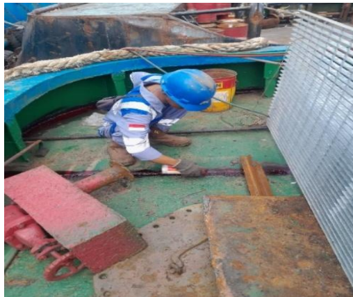
Gambar 3.78 Penetrant test TB. GONAYA 10
