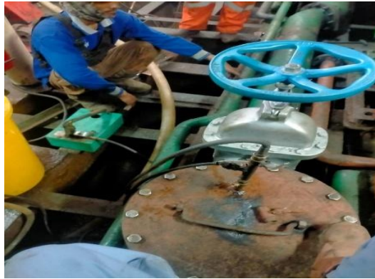
3.55 hydro test valave KMP JAMBO XI
