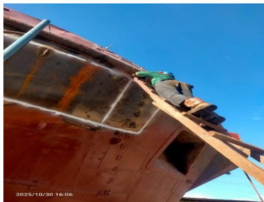
Gambar 3.83 Penetrant test TB.KSA 09
