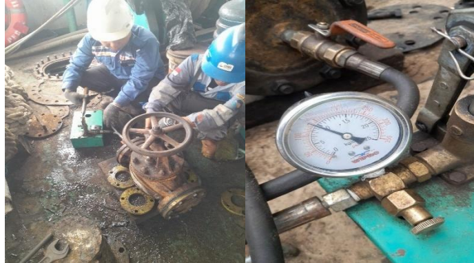
Gambar 3.17 Hydro Test Valve ME
