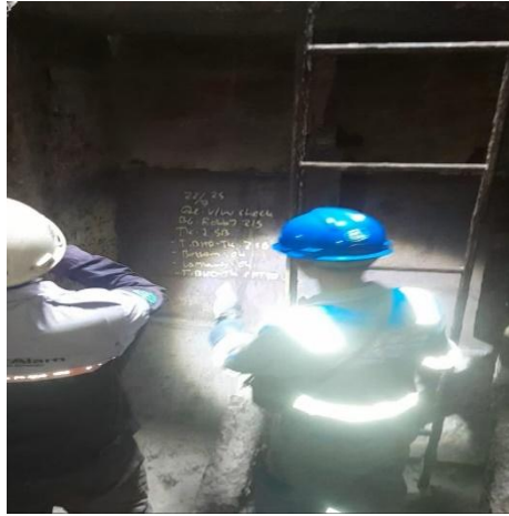
Gambar 3.2 inspection welding BG Robby 215
