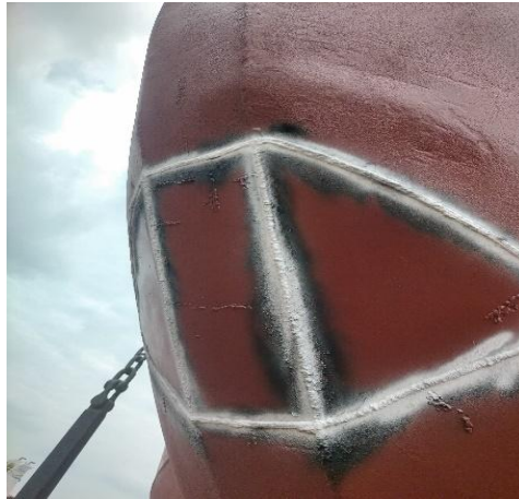
Gambar 3.18 Penetrant test Bulbous Bow
