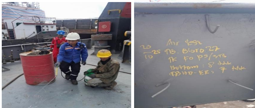
Gambar 3.75 Proses Air Test Tb.Bloro 27
