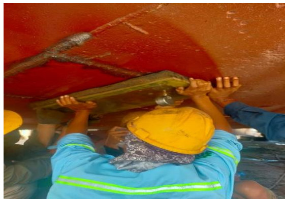
Gambar 3.57 vakum test TB.KSA 18
