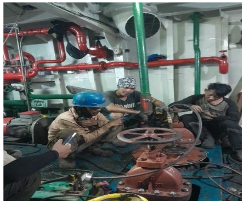
Gambar 3.85 hydro test KMP.JAMBO VIII
