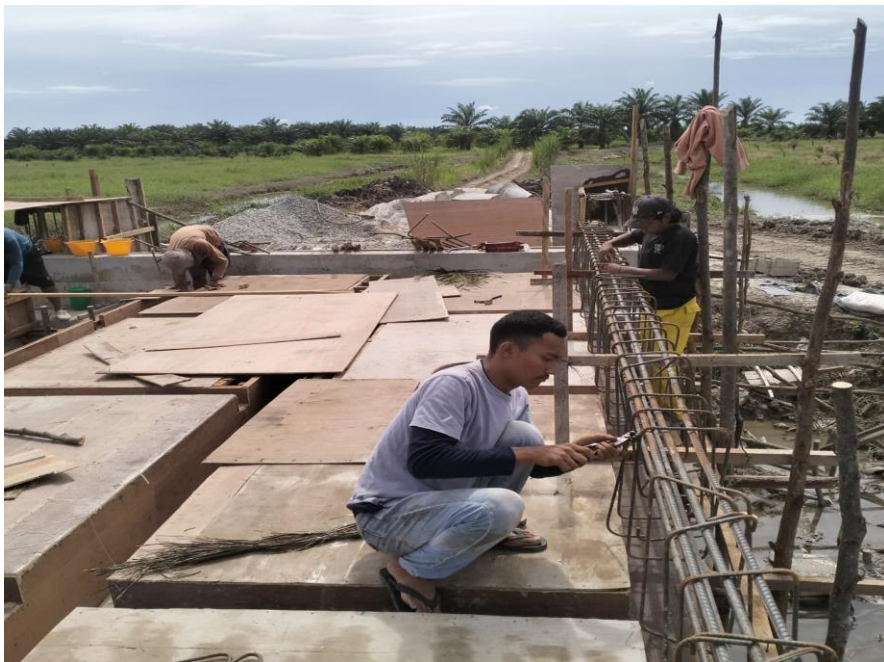
Proses Perakitan Besi Girder & Diafragma
