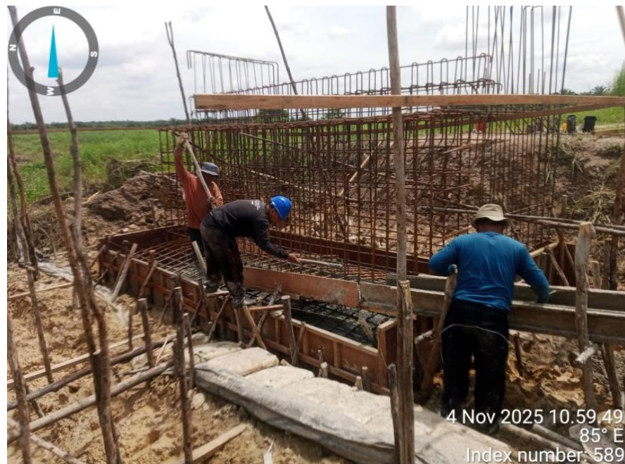
Proses Pengecoran Pile Cap
