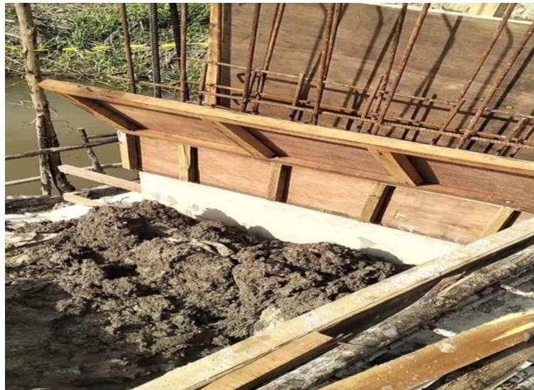
Gambar 3.35 Proses Pengecoran Sayap Abutment
