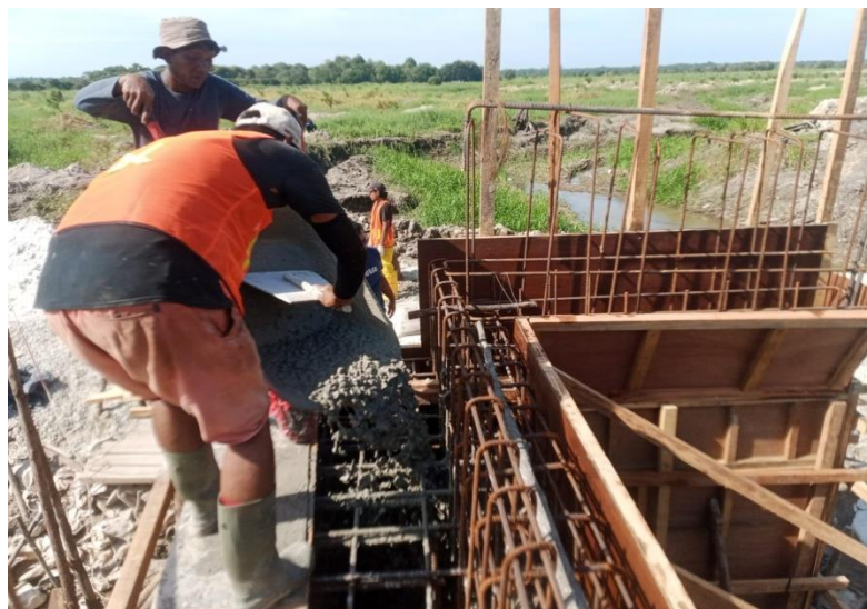
Gambar 3.28 Proses Pengecoran Tiang Abutment
