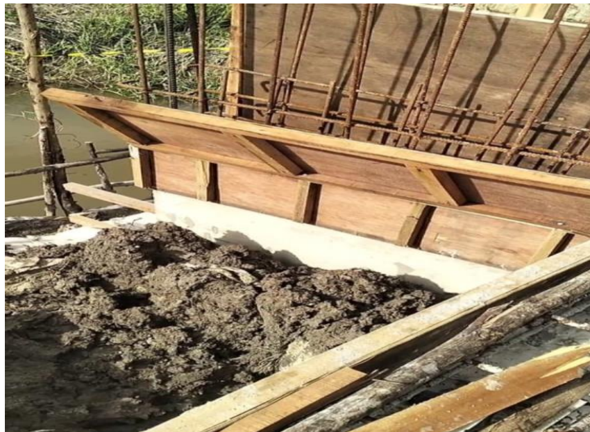
Proses Pengecoran Wing Wall
