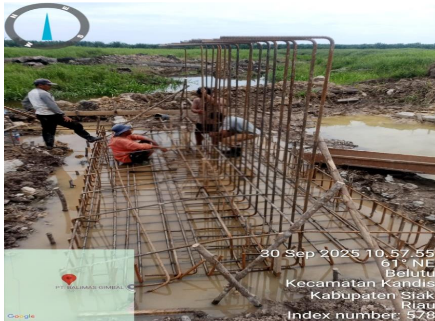
Proses Perakitan Besi Stem Wall & Wing Wall
