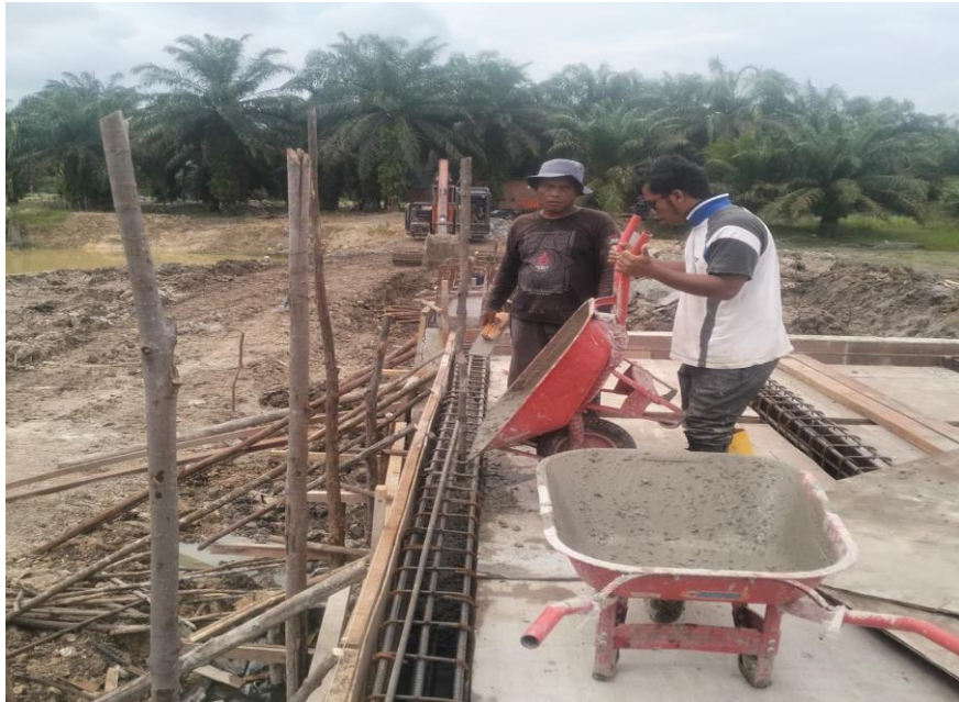
Proses Pengecoran Balok Girder
