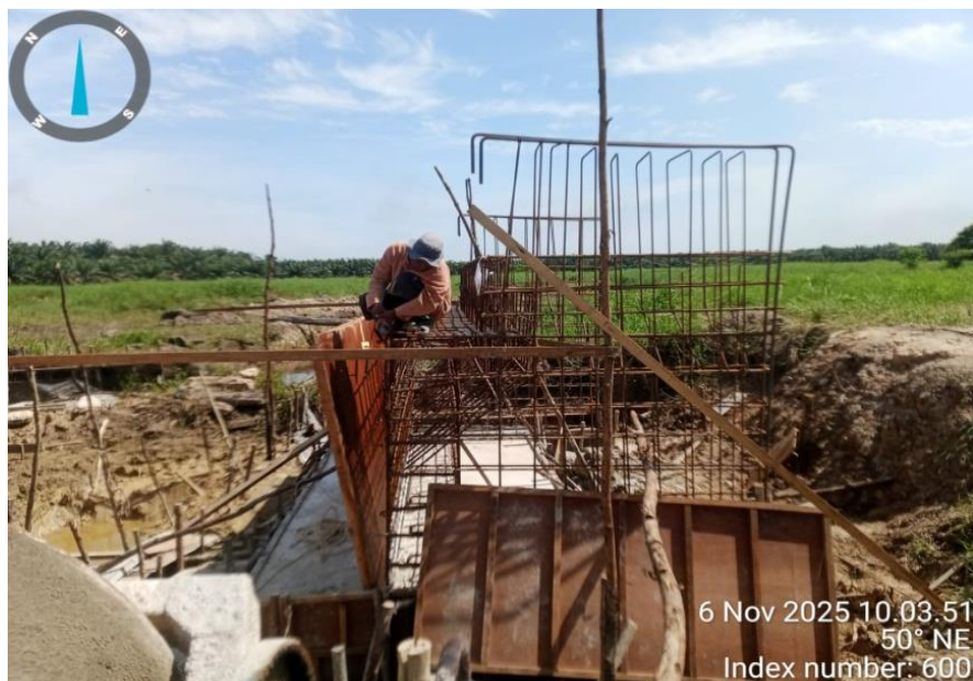
Proses Perakitan Mal Stem Wall & Wing Wall
