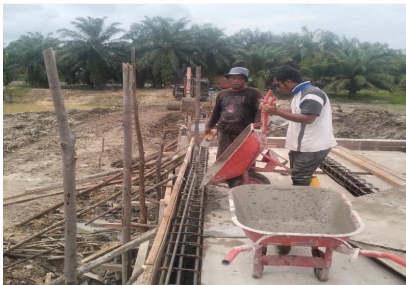
Gambar 3.32 Proses Pengecoran Balok Girder
