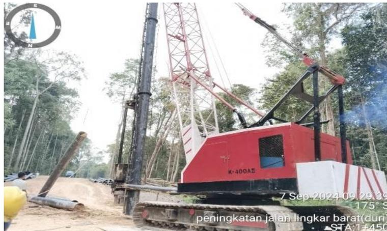
Gambar 3. 7 Diesel hammer
