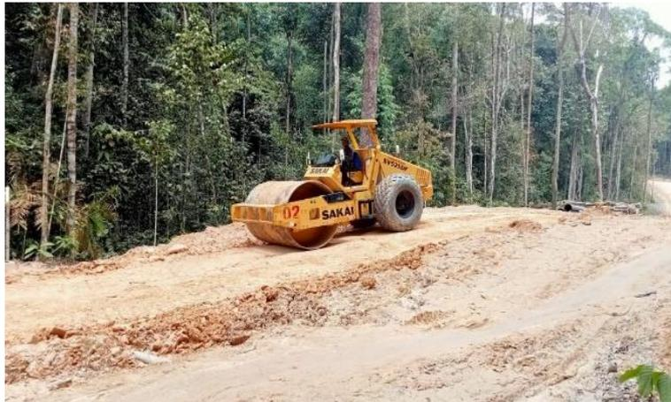
Gambar 3. 5 Vibration roller
