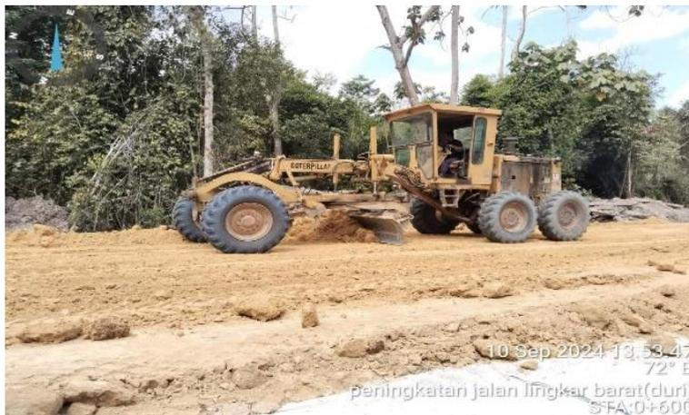
Gambar 3. 4 Motor grader
