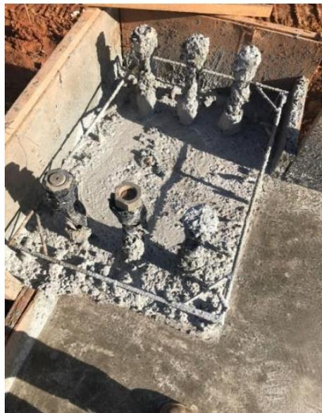
Gambar 3. 24 Pemasangan Bekisting *Equipment*
