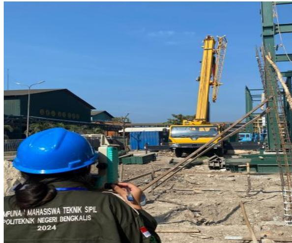
Gambar 3. 33 Mengecek *Verticality* Kolom
