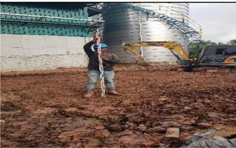
Kontrol elevasi slab concrete floor extraction
