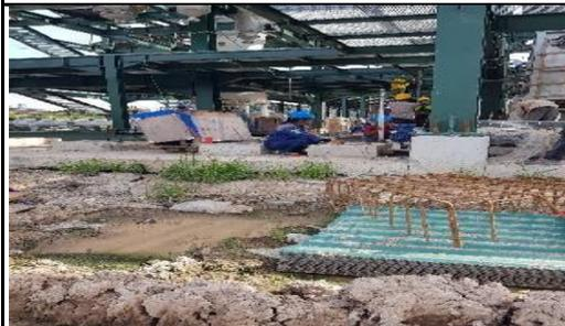
Marking elevasi baut dududan pondasi equipment di extraction plant
