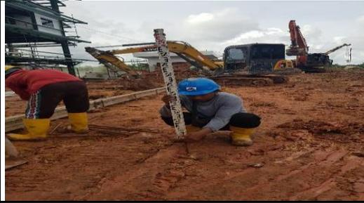
Cek elevasi bekisting slab concrete floor extraction
