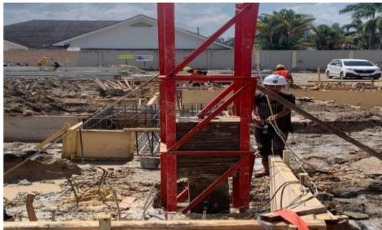
Gambar 3. 16 *PDA Test*
