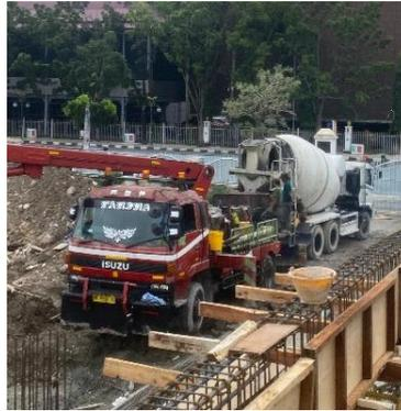
Gambar 2. 21 Concrete pump
