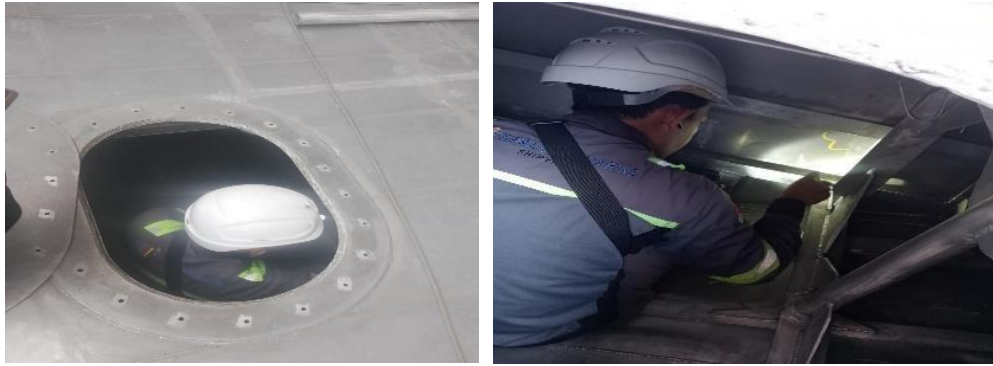
Gambar 3.28 pengecekan welding pada aft peak tank
