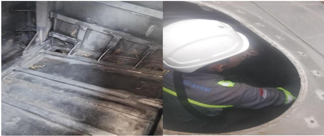
Gambar 3.27 pengecekan welding aft peak tank
