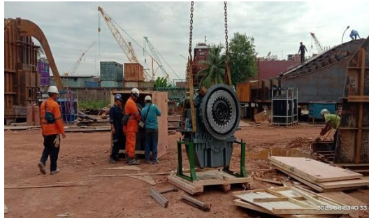
Gambar 3. 57 Erection Gearbox
