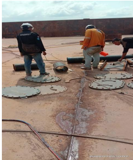
Gambar 3. 20 External air pressure test
