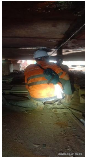
Gambar 3. 34 Proses Air Pressure Test Eksternal
