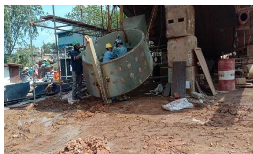
Gambar 3. 33 proses Erection Kort Nozzle
