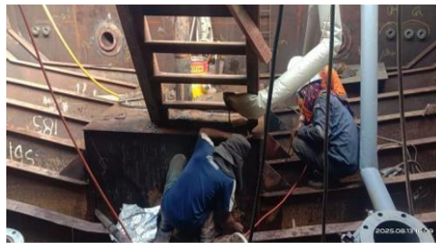
Gambar 3. 50 Air Pressure Test eksternal tangki ( LOT )
