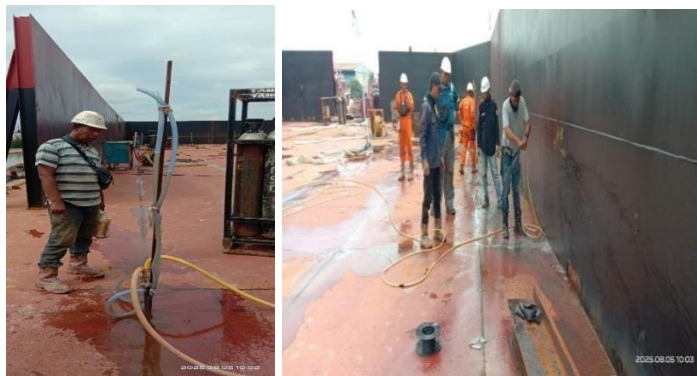
Gambar 3. 37 Air Preasure Test
