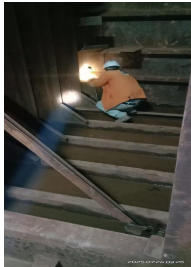
Gambar 3. 19 Visual Welding Inspection tangki
