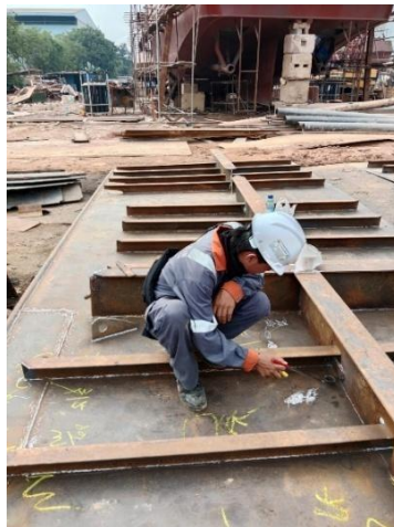
Gambar 3. 3 Visual Welding Inspection
