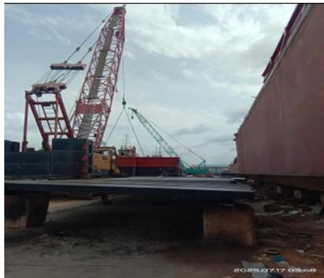
Gambar 3. 7 Proses Erection Panel Side Board
