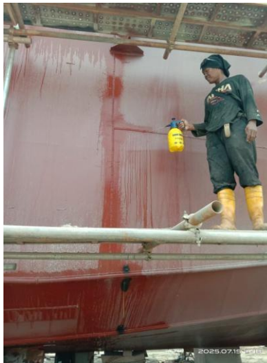
Gambar 3. 4 External Air Test
