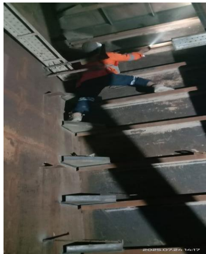
Gambar 3. 21 Visual Welding Inspection tangki
