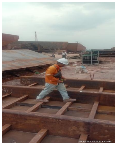
Gambar 3. 18 Inspeksi panel Main Deck
