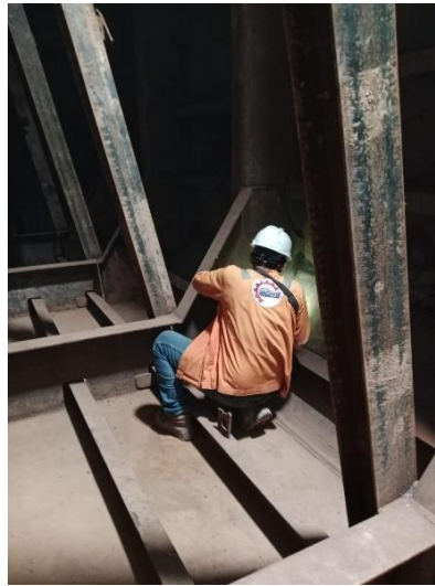
Gambar 3. 22 Visual Welding Inspection tangki
