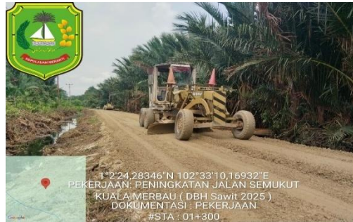
Gambar 3. 13 Penghamparan Agregat Quarry Waste
