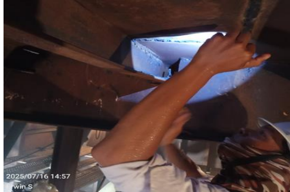
Gambar 3. 6 Welding Inspect Area Tangki Tongkang
