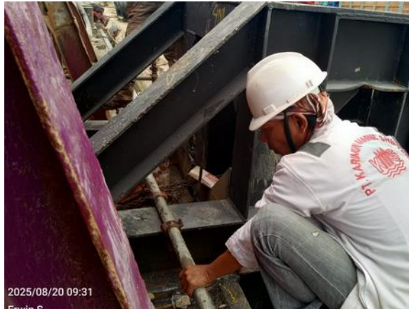
Gambar 3. 48 Welding Inspect Housing Spud Canyon
