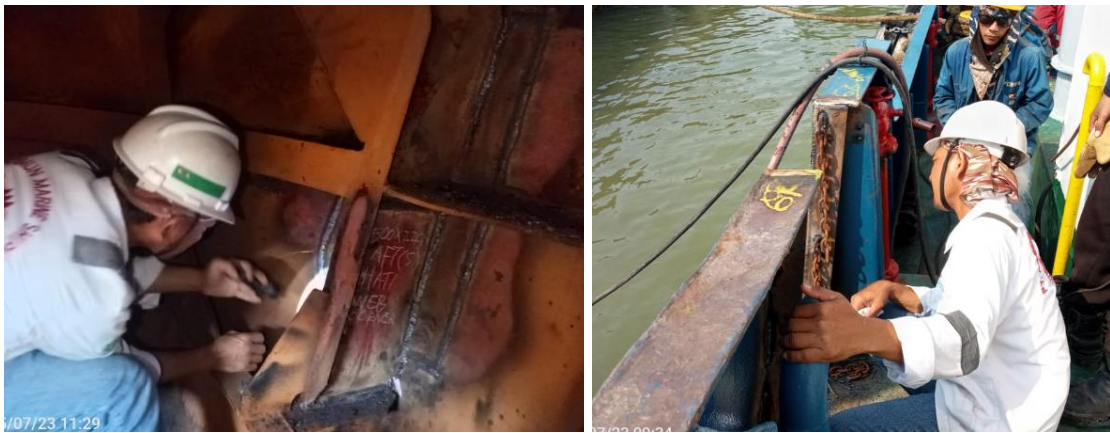
Gambar 3. 17 Welding Inspect Engine Room Dan Akse Bulk Wark
