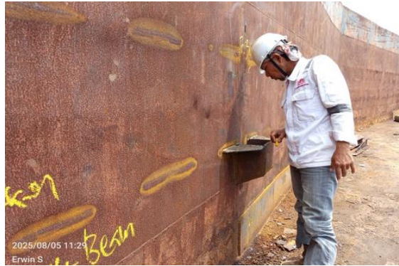
Gambar 3. 33 Welding Inspect Riper Tongkang SA995
