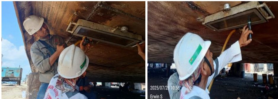
Gambar 3. 23 Vacuum Test Lintas Bahari
