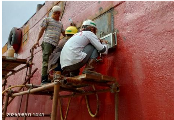
Gambar 3. 29 Uji Kebocoran Metode Vacuum
