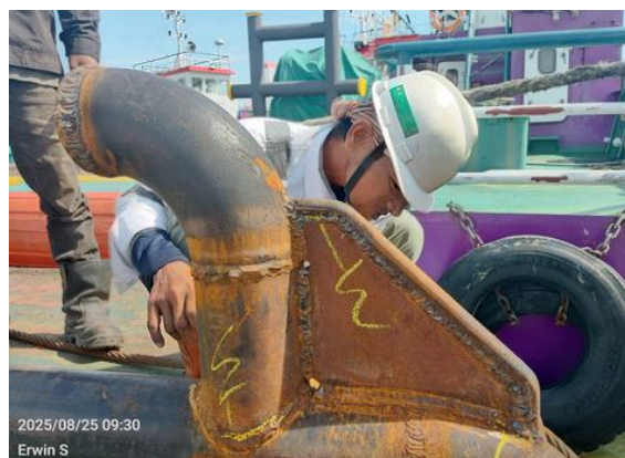
Gambar 3. 52 Welding Inspect Bracket
