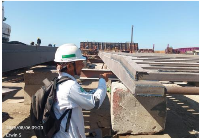
Gambar 3. 34 Welding Inspect Ramdoor Portable
