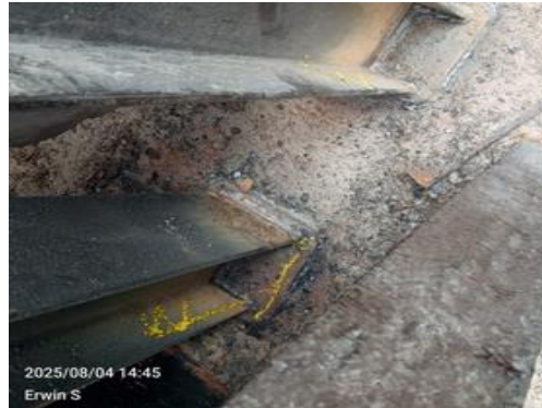
Gambar 4. 1 Welding Inspeck Extended
