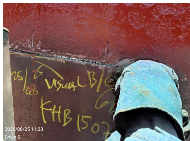
Gambar 3. 54 Welding Inspect dan Back Guaging
