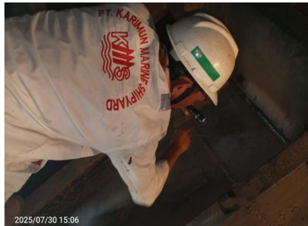
Gambar 3. 36 Welding Inspect Insert Plat Inner bootom
