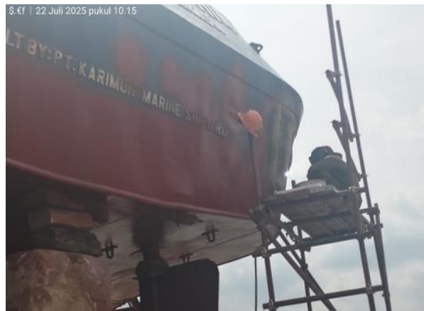
Gambar 3. 16 Welding Inspect, Insert Plat Santiago
