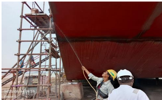
Gambar 4. 5 Proses Air Test
