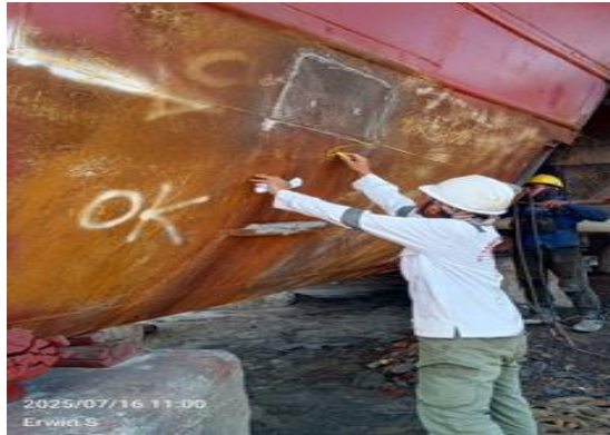
Gambar 3. 7 Welding Inspect After Capping
