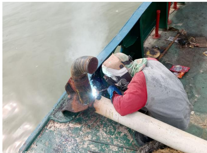
Gambar 3. 41 Welding Inspect Safety towing
