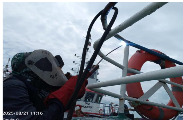
Gambar 3. 57 Visual Weld railing
