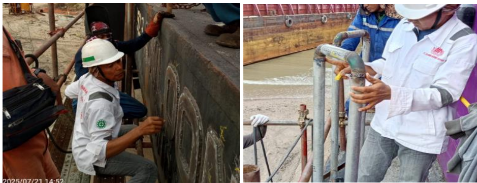
Gambar 3. 14 Welding Inspect Ship Name dan Railing
