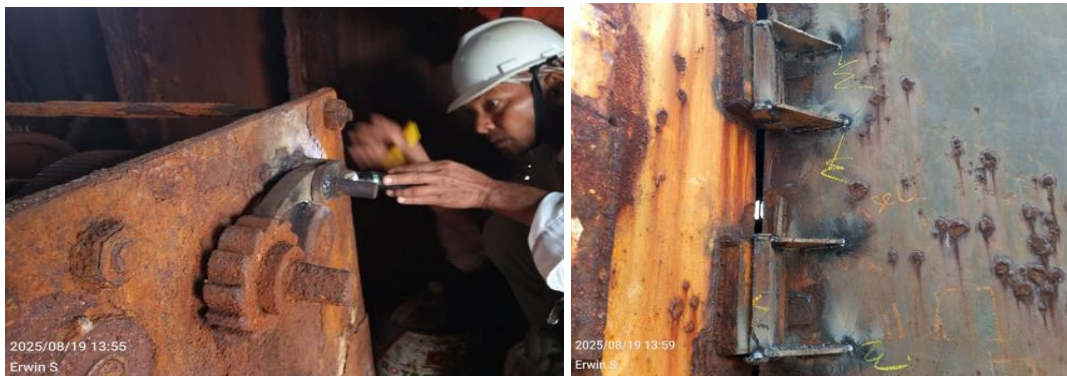
Gambar 3. 46 Welding Inspect Riper SA995
