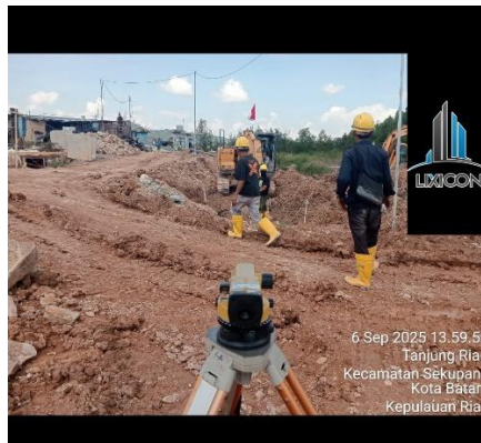
Gambar 3. 4 Leveling Top concrete
