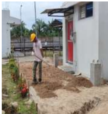
Gambar 59 Proses Penimbunan Jalan Shelter Security
