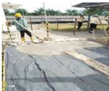
Gambar 74 Proses Pengecoran Jalan Shelter Security
