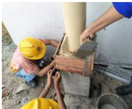
Gambar 115 Pekerjaan Grouting Kolom Pedestal Di Shalter Security
