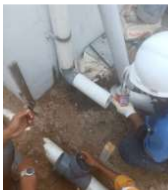
Gambar 67 Connecting Pipa Air Hujan
