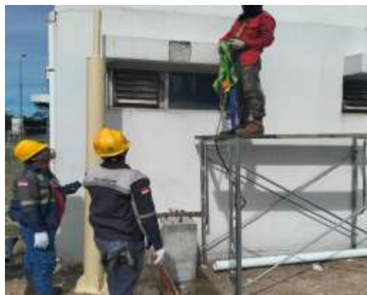
Gambar 64 Proses Erection Tiang Knopi
