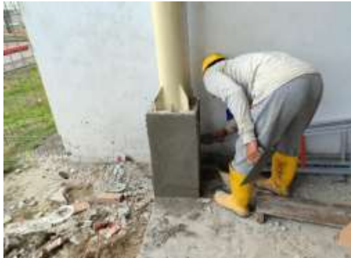
Gambar 125 Pekerjaan Acian Kolom Pedestal Di Shelter Security
