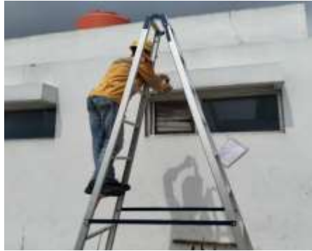
Gambar 39 Proses Making Pembobokan Tiang
