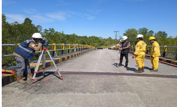
Gambar 3 . 2 Survey stake out
