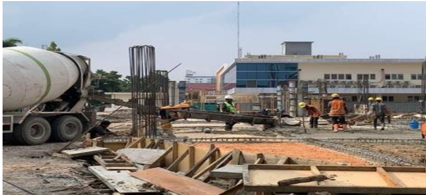
Gambar 3. 64 Beton Ready Mix
