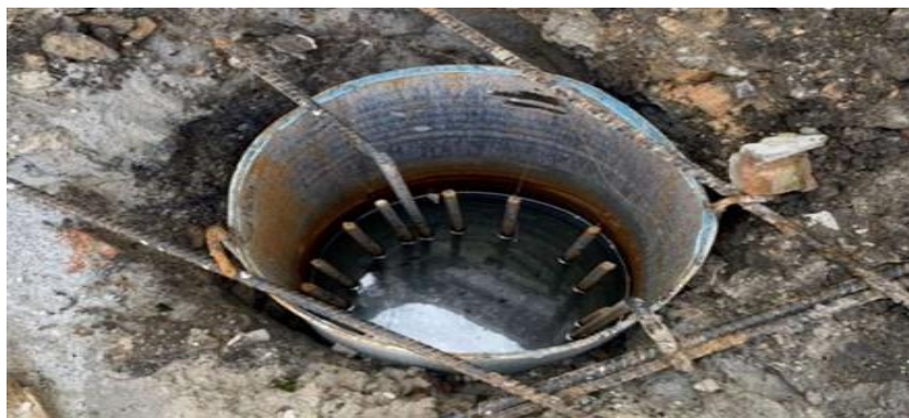
Gambar 3. 14 Pondasi Bore Pile
