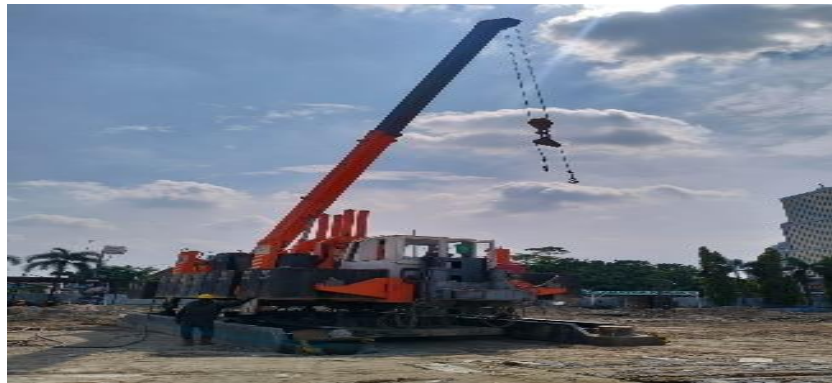
Gambar 3. 74 HSDP ( Hidrolic Static Pile Driver )
