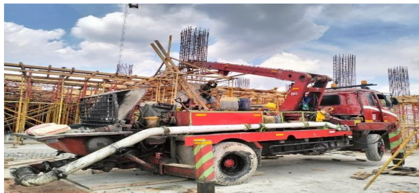
Gambar 3. 75 Concret pump
