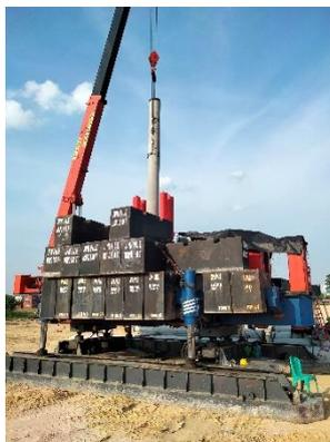
**Gambar 3. 2** Hydraulic static pile driver (HSPD)
