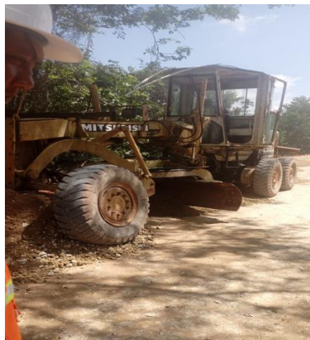
Gambar 3. 12 Perataan agregat base B
