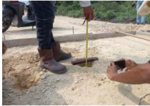
Gambar 3. 16 Pengukuran Test Pit Base B
