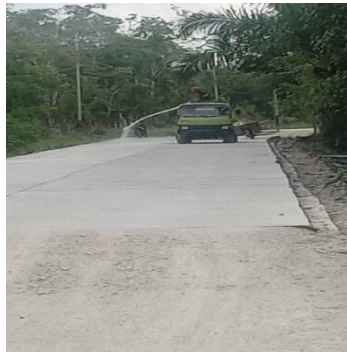
Gambar 3. 34 Pekerjaan Curing Compound
