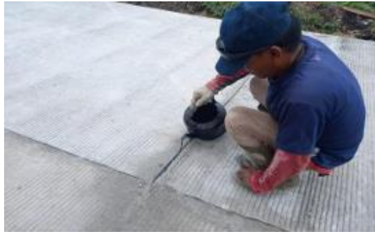
Gambar 3. 36 Pekerjaan Joint Sealent
