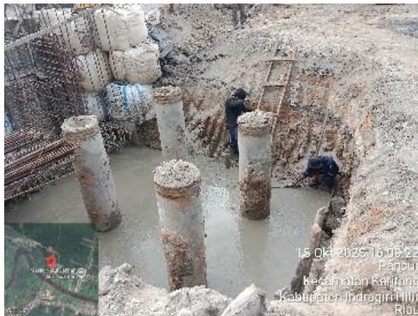
Gambar 3. 44 Pengecoran Lean Concrete
