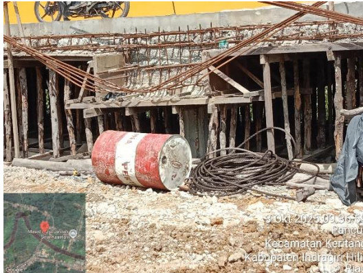
Gambar 3. 19 Bahan Bakar Diesel (Solar)
