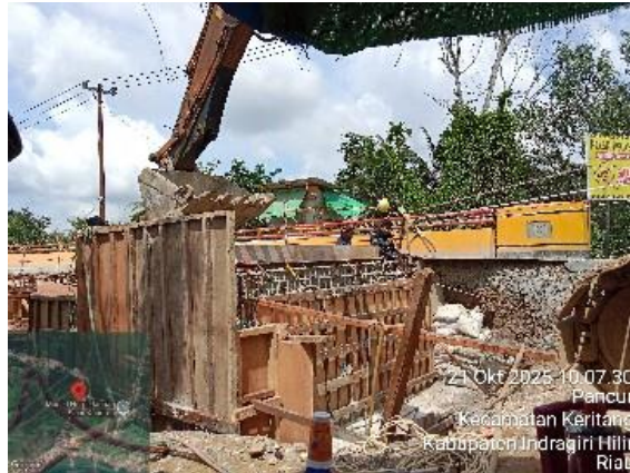
Gambar 3. 47 Pengecoran abutment
