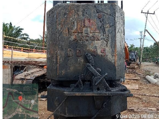
Gambar 3. 24 Diesel Hammer
