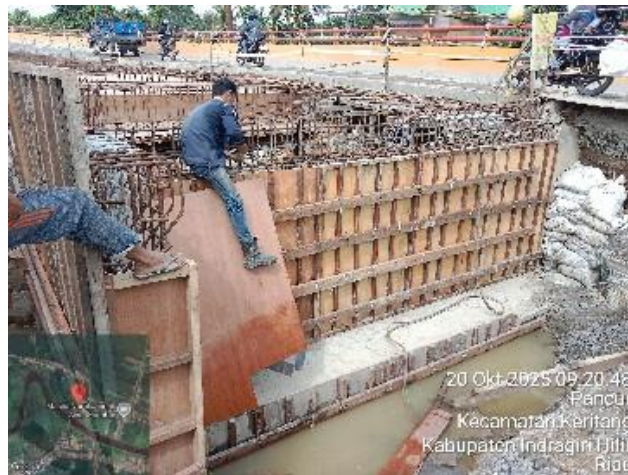
Gambar 3. 46 Pemasangan bekisting abutment
