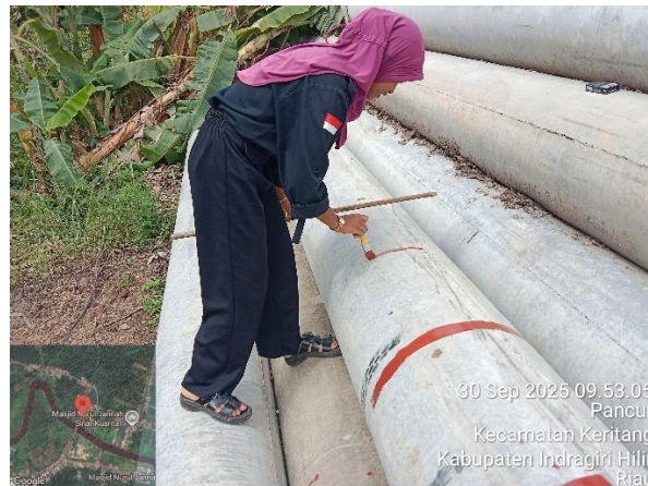
Gambar 3. 5 Penandaan spun pile
