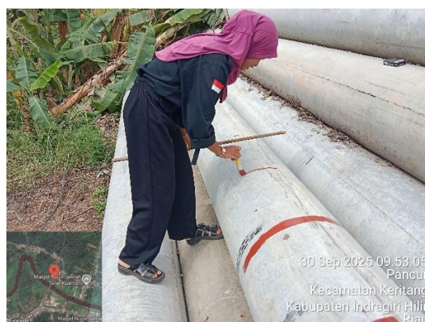
Gambar 3. 32 Penandaan spun pile
