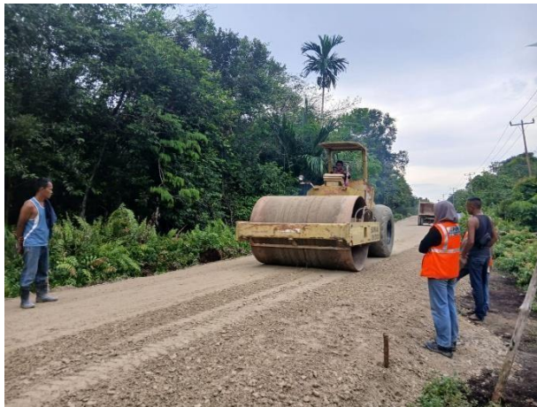
Gambar 3. 22. Pedatan quarry waste.
