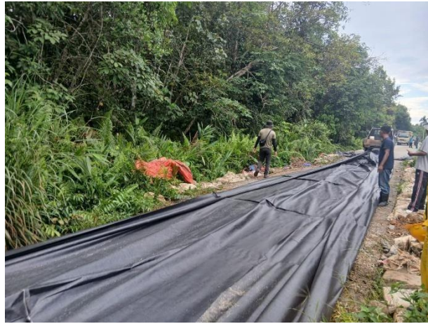
Gambar 3. 18.Pemasangan Geotextile
