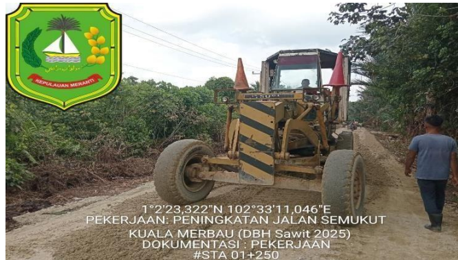
Gambar 3. 13 Motor Grader
