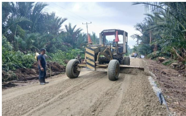
Gambar 3. 21. Perataan quarry waste
