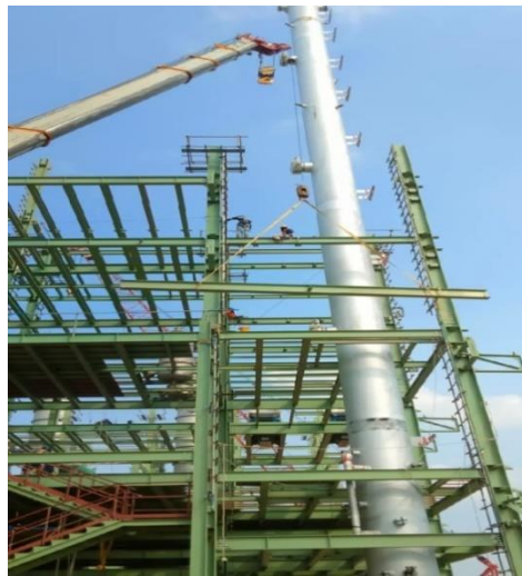
Gambar 3.7 erection main beam
