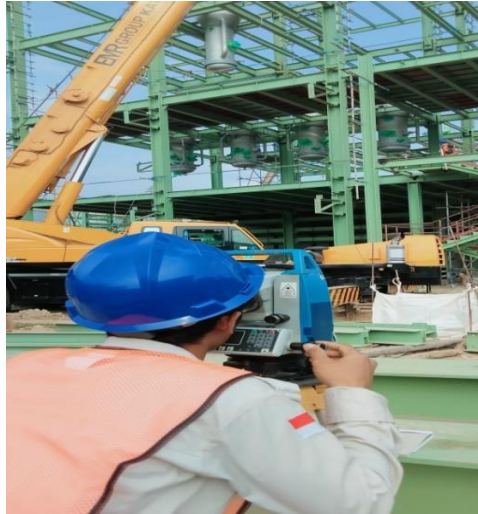
Gambar 3.11 verticality kolom
