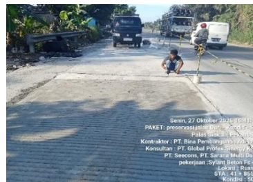
Gambar 3. 49 joint sealant (Sumber Dokumentasi Lapangan 2025)
