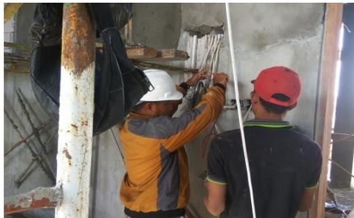
Gambar 3. 61 Instalsi Stop Kontak
