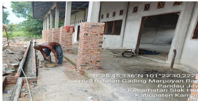
Gambar 3. 28 Plasteran Kolom Teras
