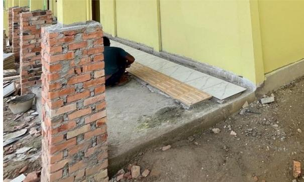
Gambar 3. 46 Pemasangan Block Dan Warning Block
