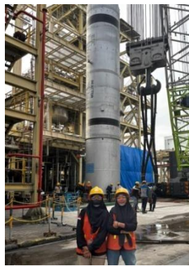
Gambar 3. 46 Lifting Vessels Reactor
