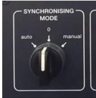
Gambar 4. 16 Selector Synchronsing Mode
