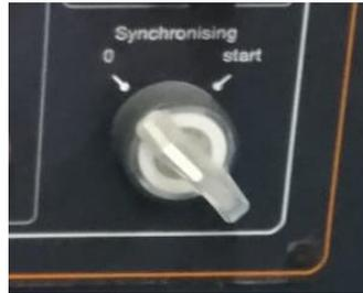
Gambar 4. 13 Selector Synchronizing CFC
