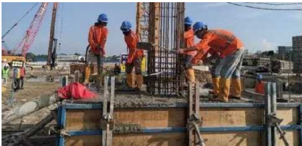
Gambar 3. 8: Pengecoran Pile Cap
