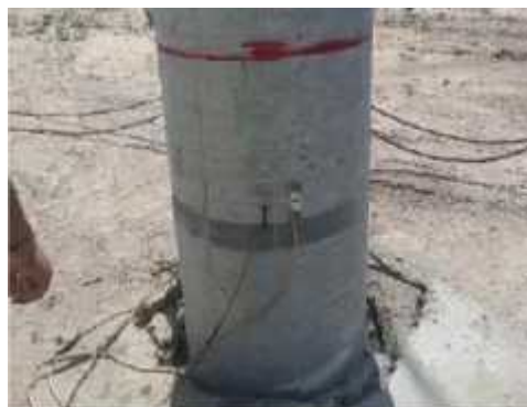
Gambar 3. 2: Penentuan Titik As Pile Cap
