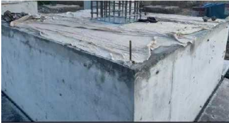
Gambar 3. 9: Proses Perawatan Beton (Curing) Pile Cap
