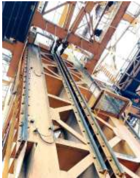
Gambar 3. 6 Lifting Sumber: PT.PLN Nusantara Power
