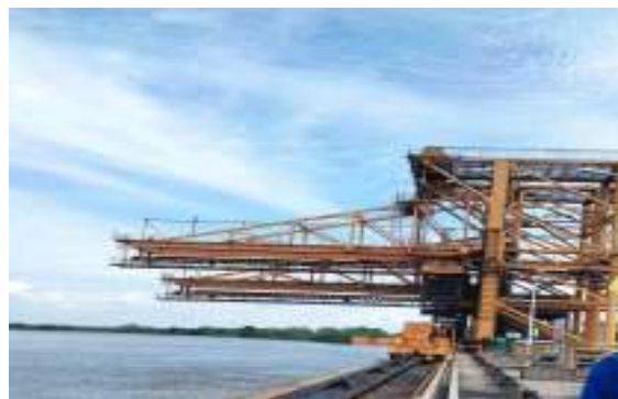
Gambar 3. 1Ship Unloader Sumber: PT.PLN Nusantara Power
