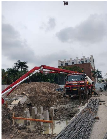
Gambar 3.19 Concrete Pump
