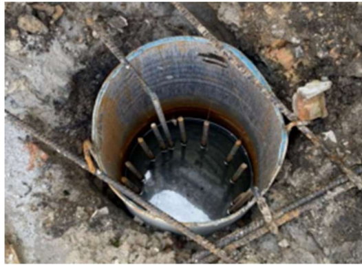
Gambar 2. 2 Pondasi Bore Pile
