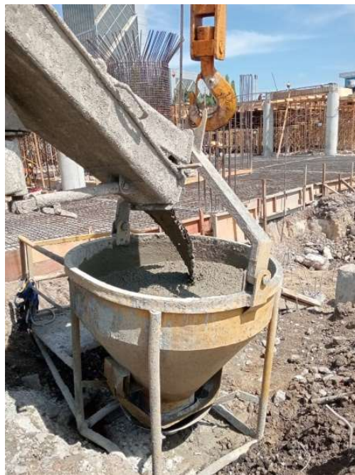
Gambar 3. 21 Beton Ready Mix
