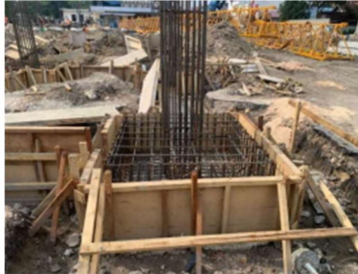
Gambar 2. 3 Pile Cap
