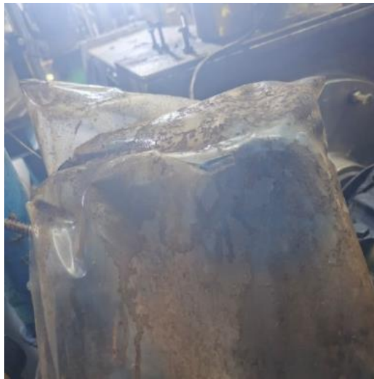
Gambar 3.6 Before Pengantian cover PVC dan pembersihan housing
