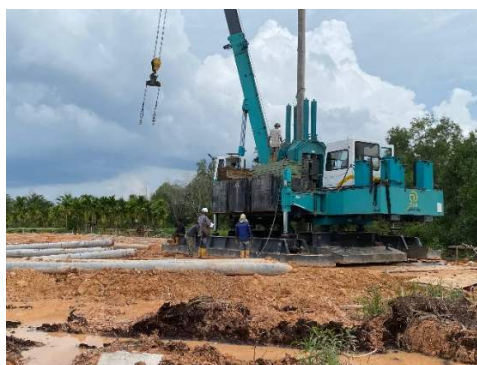
Gambar 2.12 Mesin Pancang HSPD ( Hydraulic Static Pile Driver )
