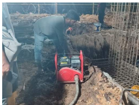
Gambar 2.22 Concrete Vibrator
