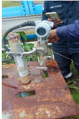
Gambar 3. 6 Differential Pressure Flow Transmitter (FIT-10) Sumber : (Dokumentasi)
