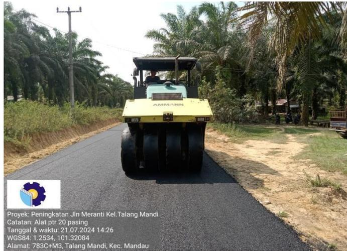
*GAMBAR 3 4 pneumatic tire roller*
