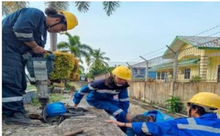
Gambar 3. 4penggantian line pipa air 2 inch
